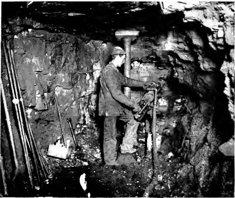
THE BREAST OF A TUNNEL, 1500 FT. BELOW THE SURFACE.
